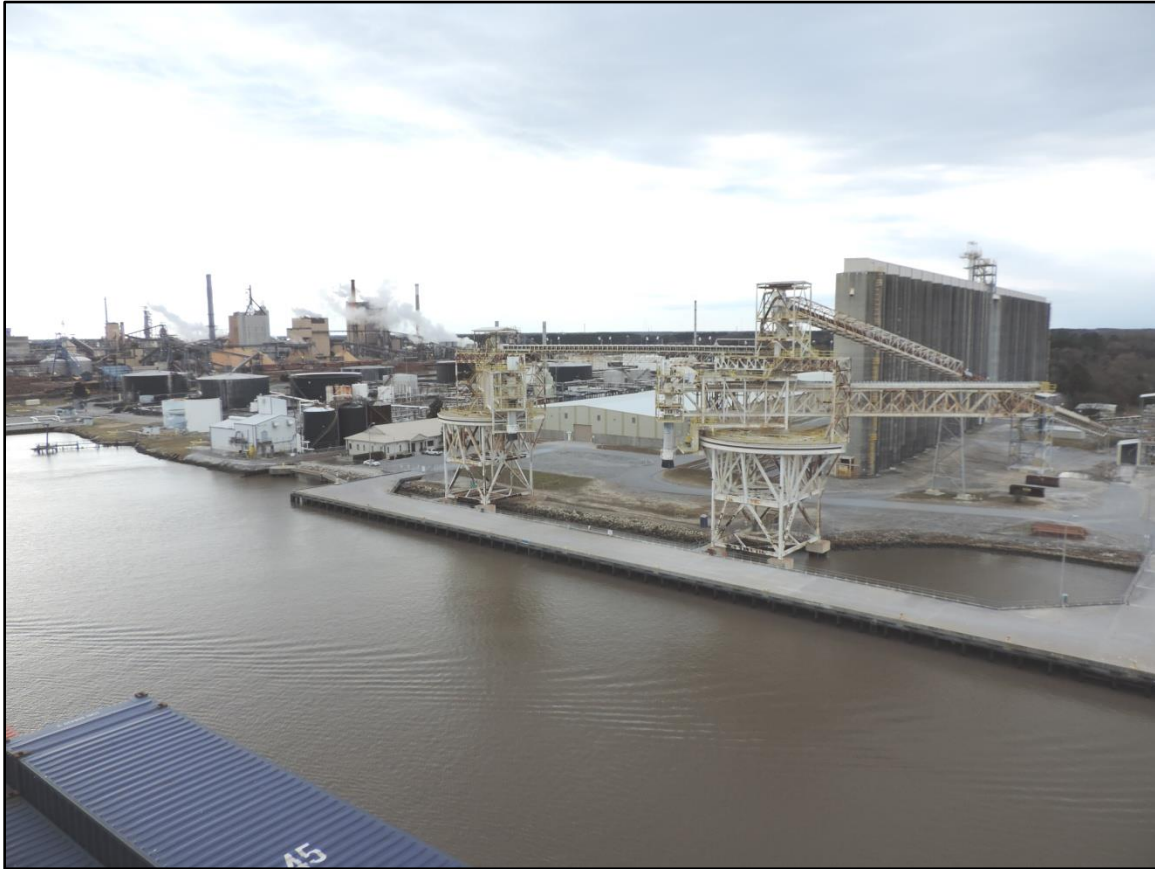
Colonial Oil Terminal Plant 3
