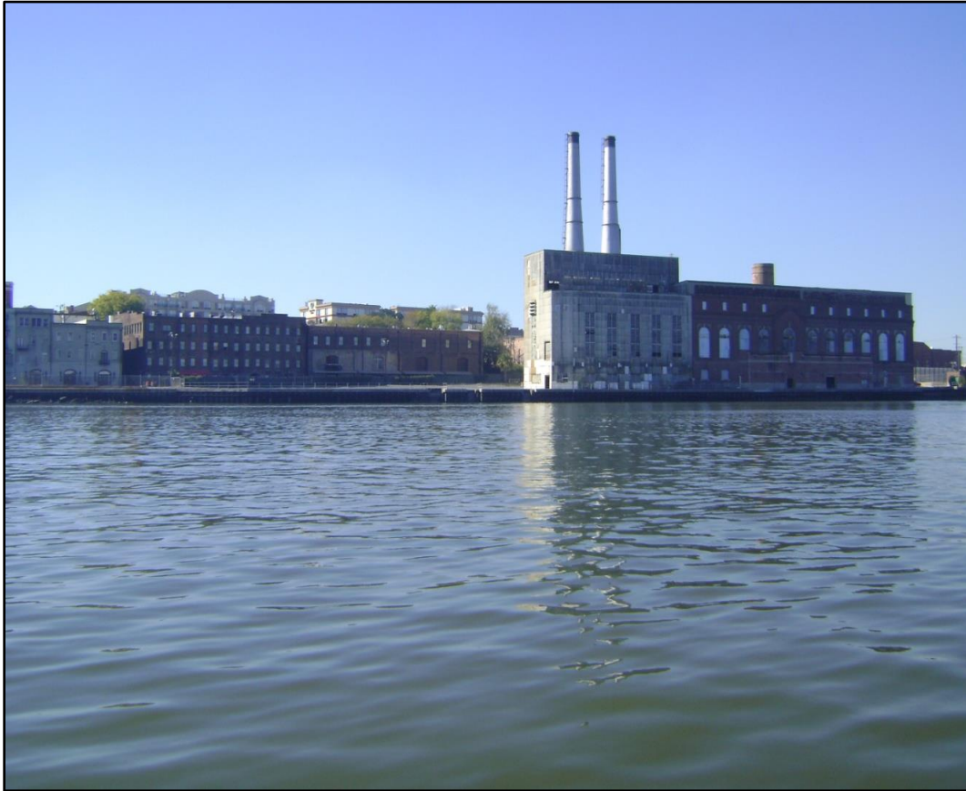
After recent demolition work
