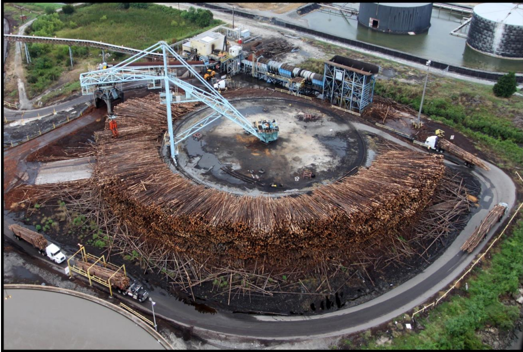
Logs dropped in the hopper – within an about 3 hours, will become paper
