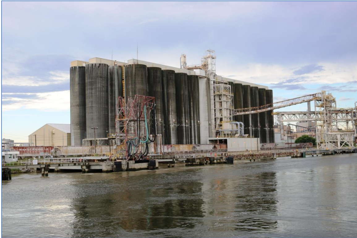
One of two kaolin silos - Colonial Oil Terminal 2
