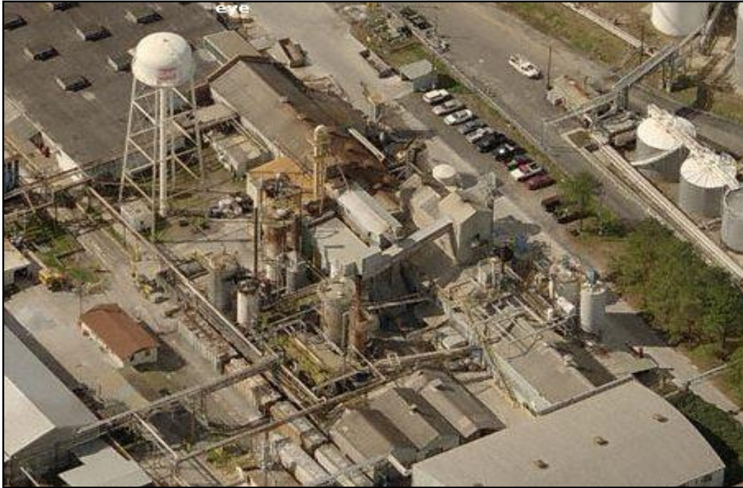
GAF water tower is visible from the river
