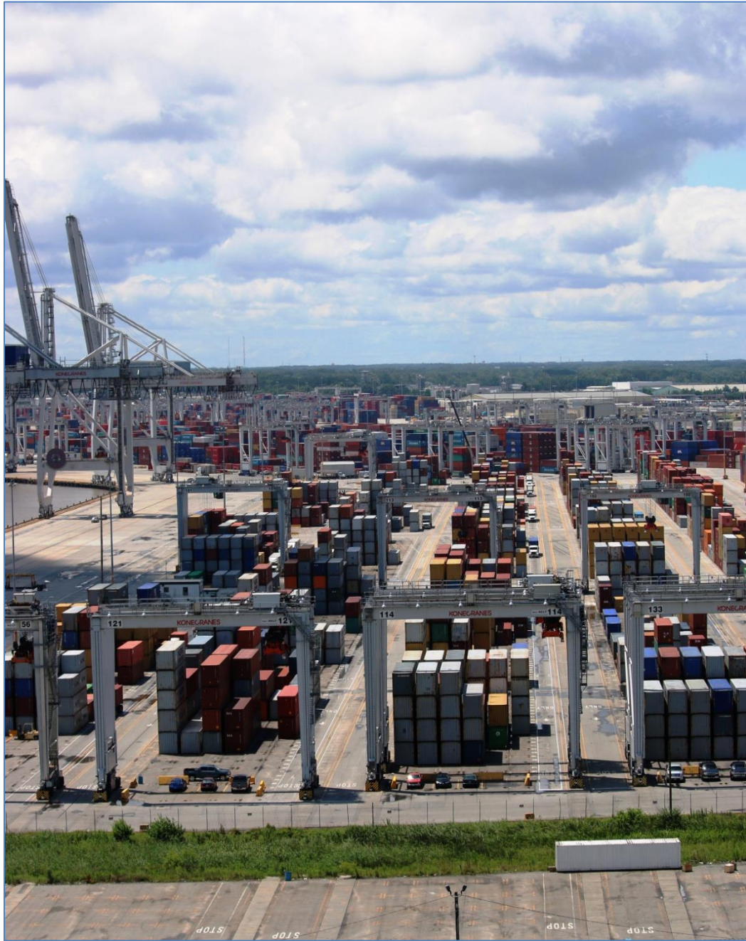
Looking southwest toward massive container yard
