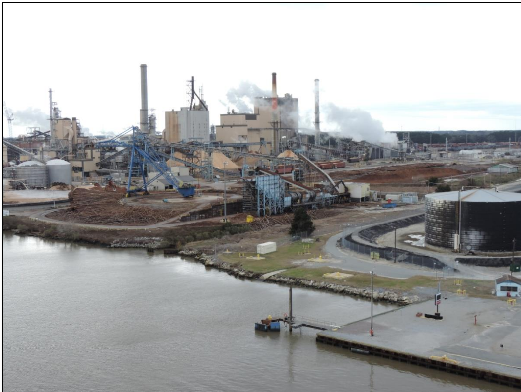
IP's wood yard with #13 power & #15 recovery boilers in the background
