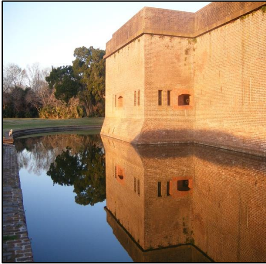
The moat surrounding the Fort
