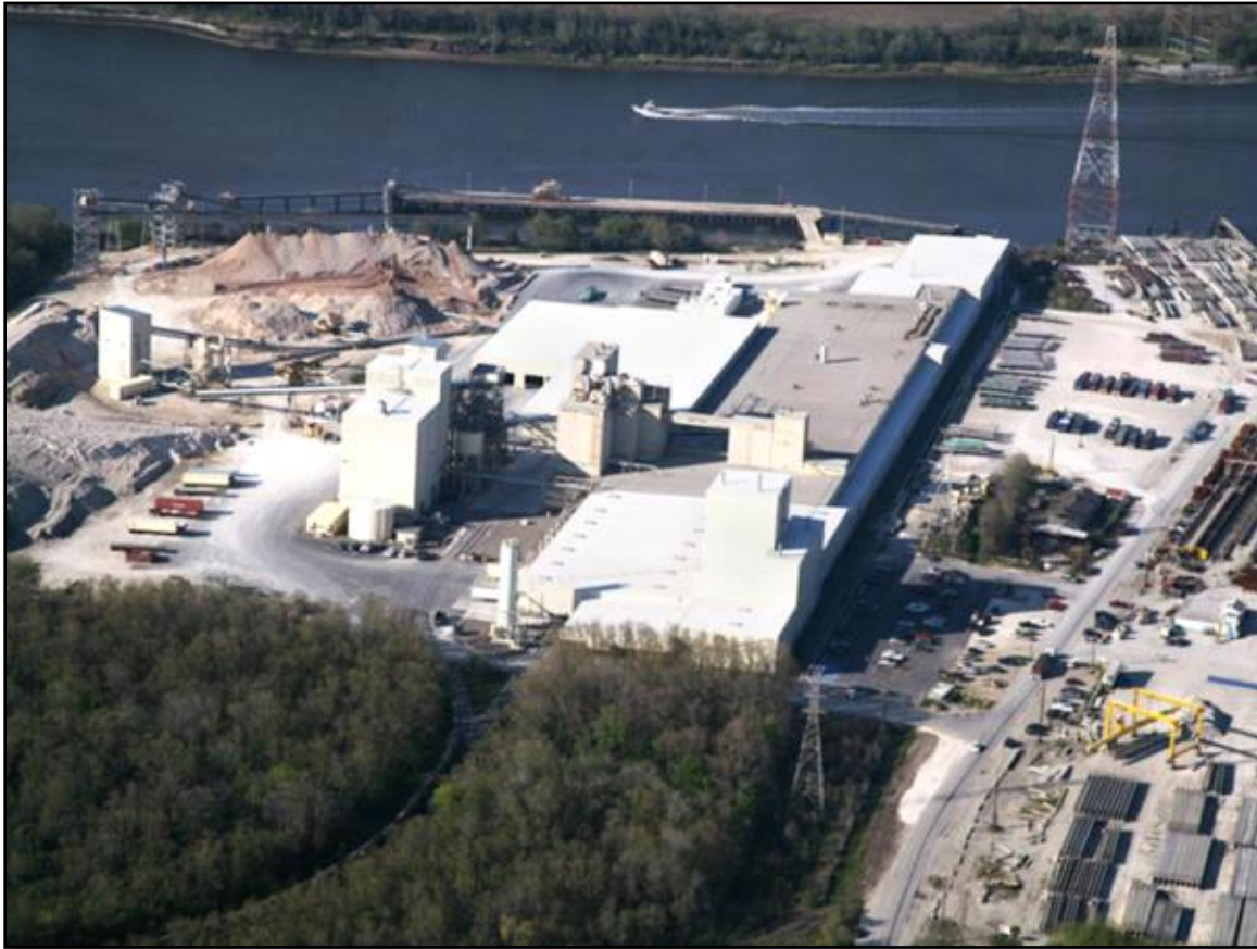
Georgia Pacific Wallboard facility
